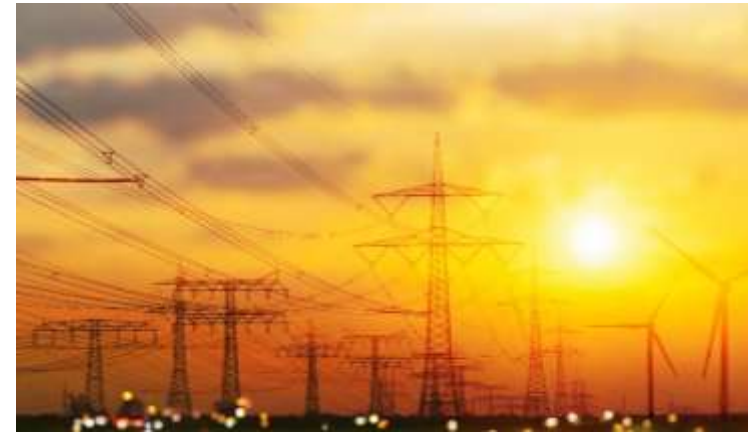
Power Network Monitoring
